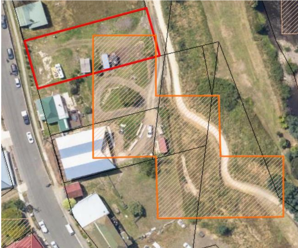
Figure 8: Aerial view of the site and the spatial extent of the landslip area shown in orange.
