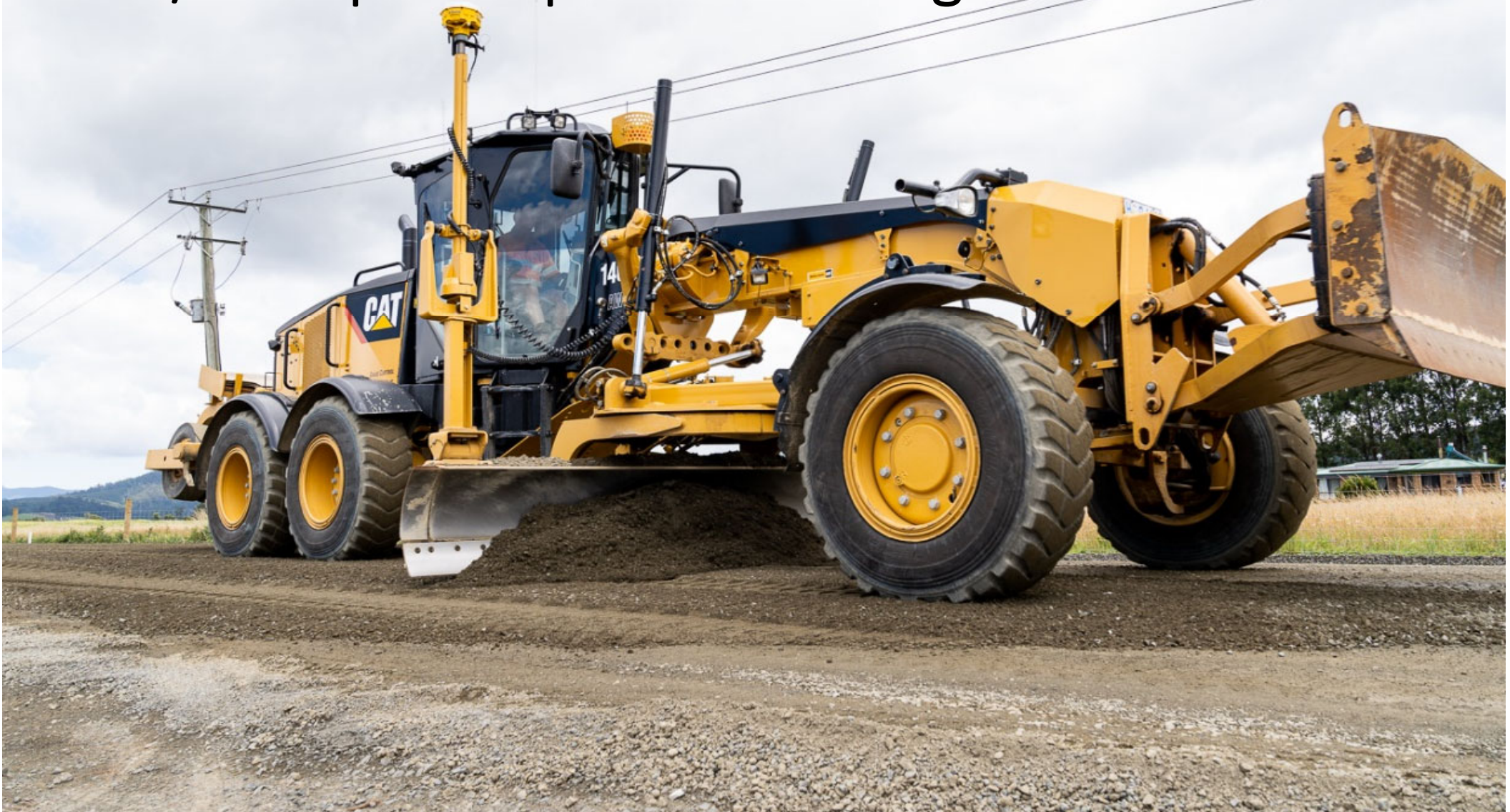
Resheeting works on Ten Mile Track, Springfield
