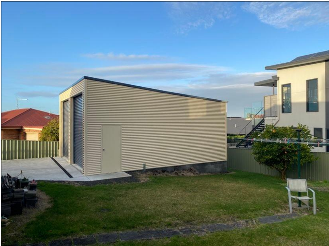
Figure 5 – Subject site, viewed from Unit 4 19 Barnett Crescent (southwestern adjoining lot), facing northeast towards the garage (photo 4pm 16 June 2023)
