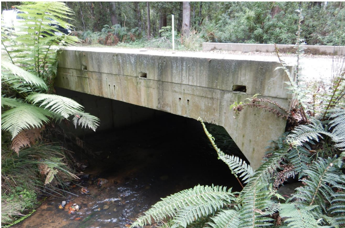
Reinforced Concrete Box Culvert 1552, Coxs Rivulet, Shanty Rd, North Scottsdale
