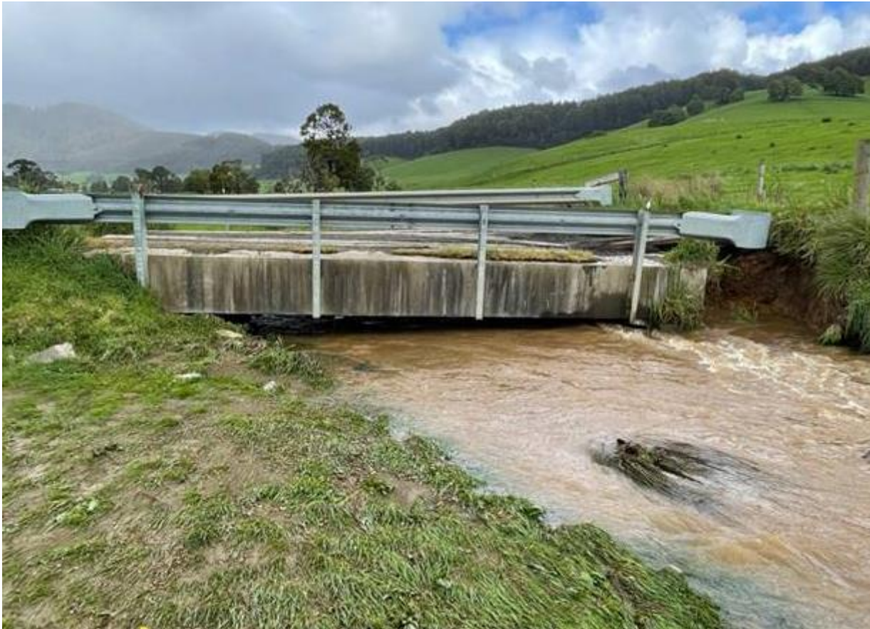
Bridge 1598 Valentine Road, Nabowla
