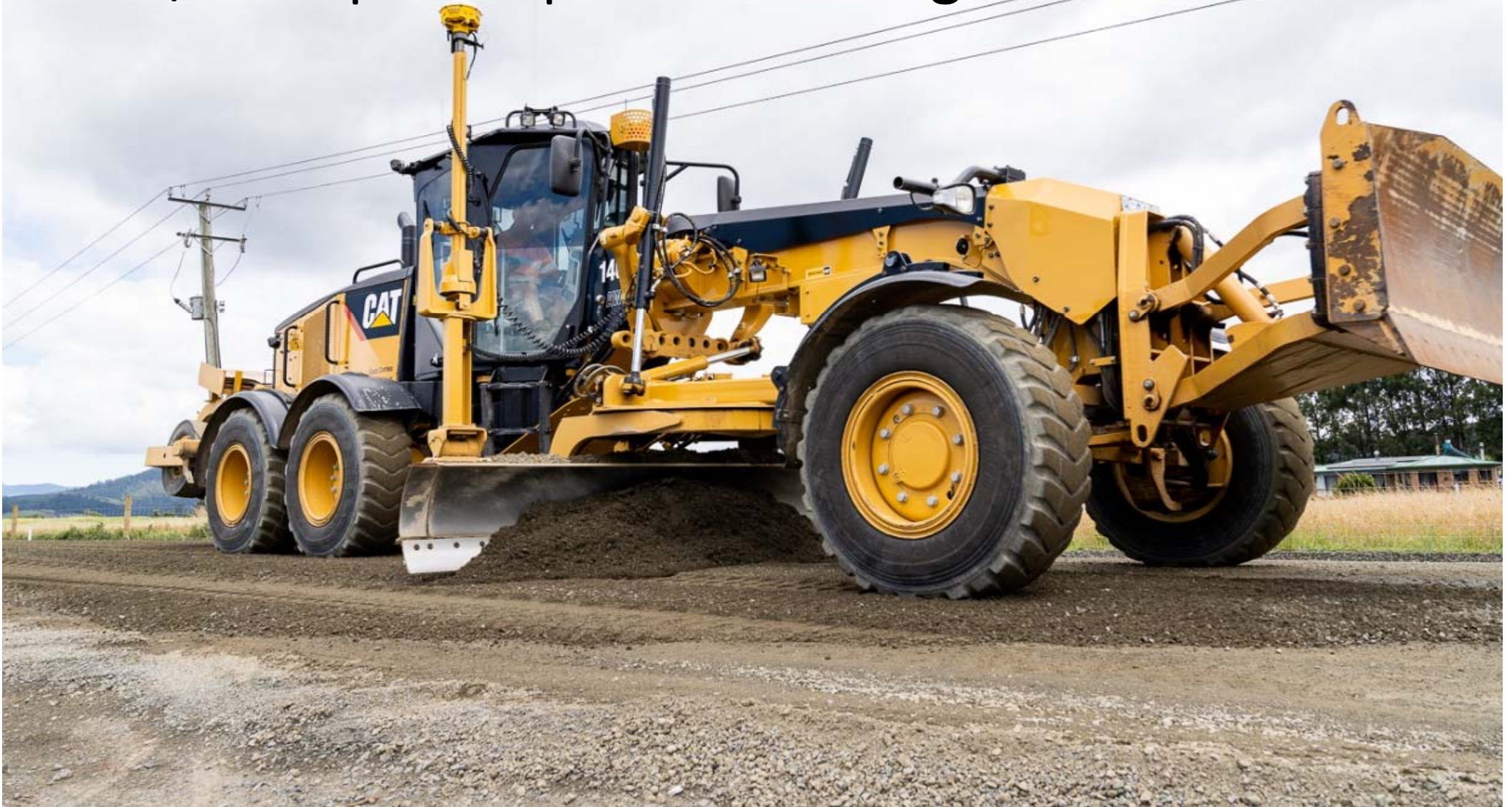
Resheeting works on Ten Mile Track, Springfield
