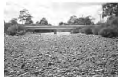
The number of piers and footings should be kept to a minimum in stream channels
