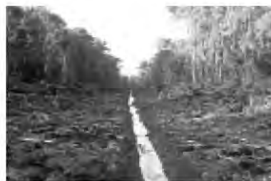
Drainage works can have significant environmental impacts
