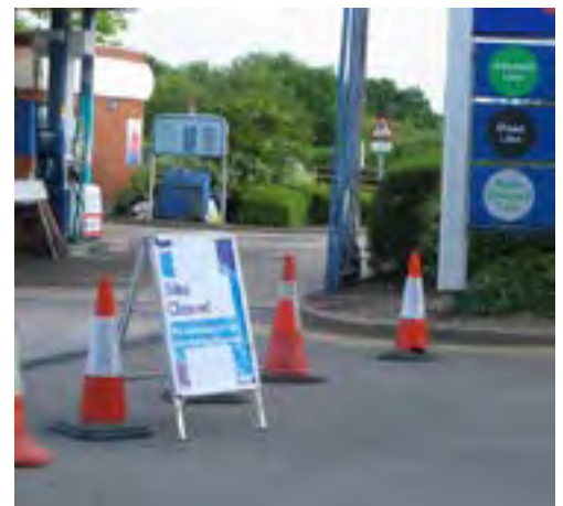
Traffic control during bulk transfer
