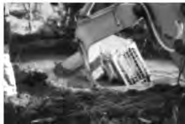
Keep machinery off wet and unstable areas
