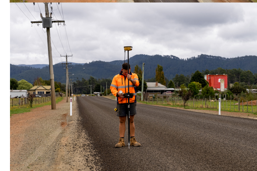
Carisbrook Lane, Legerwood | Stage 2 Reconstruction Photo Credit: NB Media
