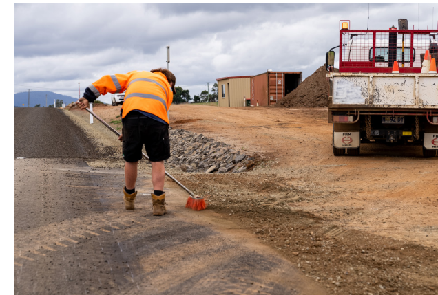
Carisbrook Lane Stage 2 Reconstruction Photo Credit: NB Media
