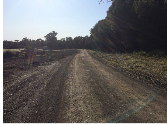
Ferny Hill Road, Golconda | Safety Improvements
