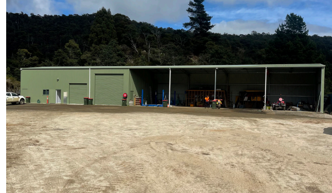
Derby Works Depot 31834 Tasman Highway DERBY
