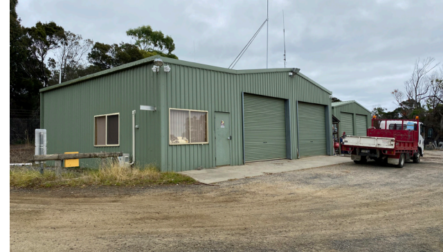
Bridport Works Depot Maxwell Street BRIDPORT
