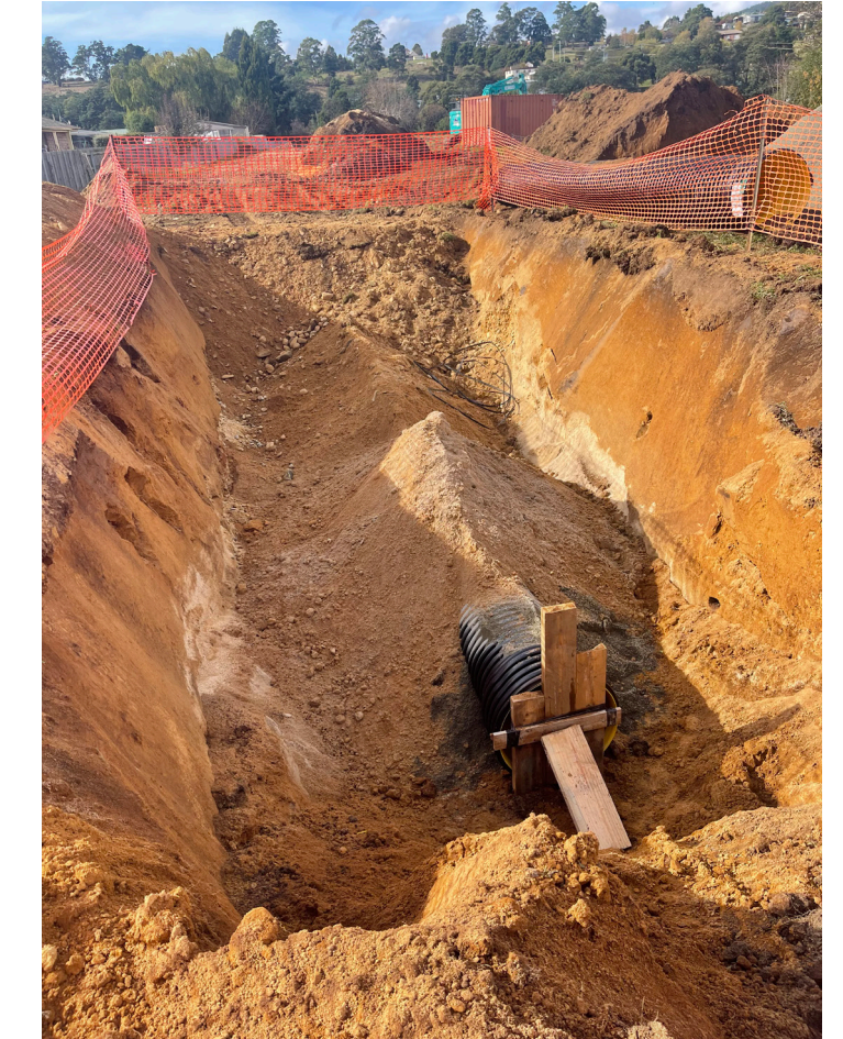
Stormwater Upgrades at Branhholm
